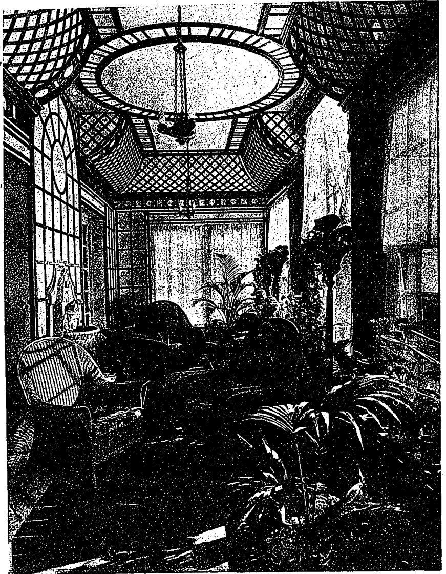
SUN ROOM, HOUSE AT WESTMOUNT, P.C.
