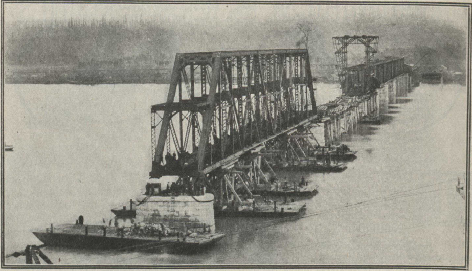
MOVING A SPAN OF THE FRASER RIVER BRIDGE
