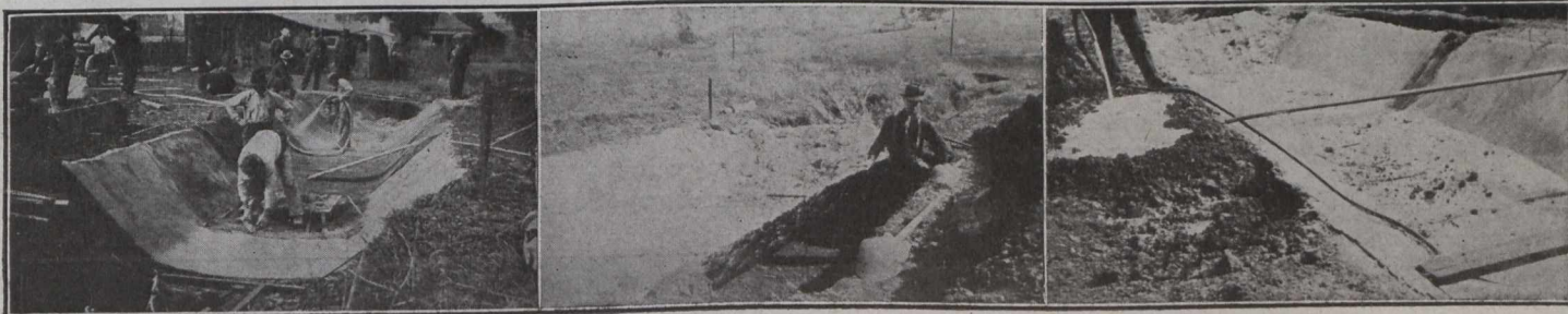
Filling Trench to Apply Hydraulic Head.
