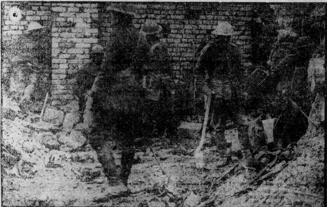
Making new dug-outs on newly captured ground. —Photo by courtesy of C. P. R.
