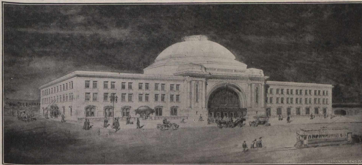
FORT GARRY STATION, WINNIPEG
