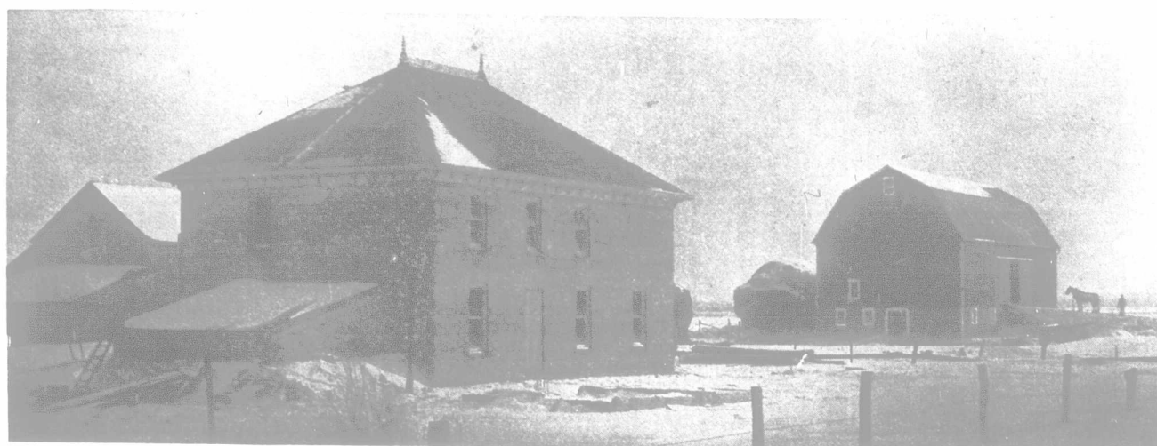
HOUSE AND BARN OF MR. J. E. REAVELEY, AT MARSHVILLE, ONT. (Size of house, 28x40x22 high. Size of barn walls, 40x80x10.)
