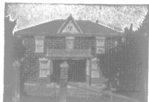
L. B. Stouffer, Plattsville, heats this large house with a Hecla that cost only $160.00 to install. He gets summer comfort for 7 tons of coal.
