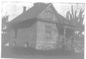
A. E. Ball's residence at Hanover, Ont. It cost just $115.00 to install a Hecla, and less than six tons of coal keeps the house comfortable all winter.
