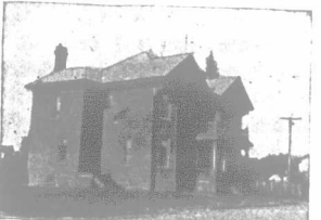
This large residence at Roseville was fitted with a Hecla Furnace at a cost of $105.00. N. B. Bricker, the owner, says he keeps it cosy with 3 1/2 tons of coal.
