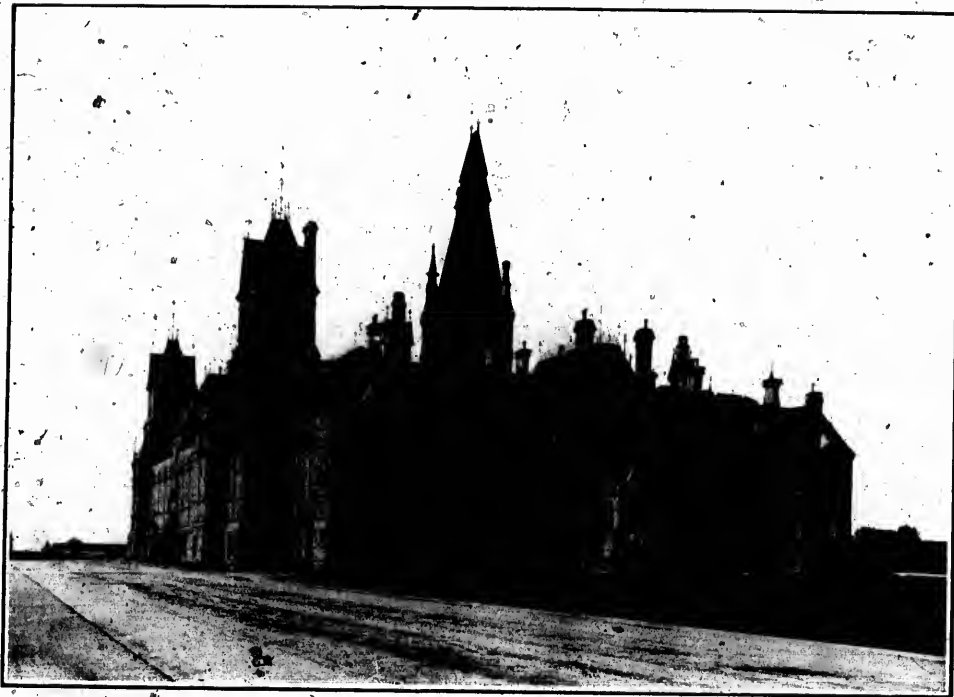
Fig. 151. —Parliament Building, Ottawa, Ontario. Fire-proofed with "Richardson's" Pressed Metal Doors, and "Hayes'" Patent Metallic Lathing.
