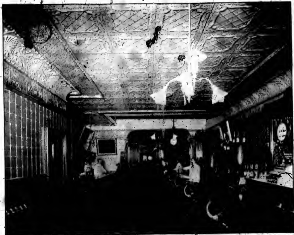
Fig. 3707. —Ceiling and Walls in Headquarters Saloon, Toronto: Plates No. 444; Mouldings No. 920; Border No. 812; Cornice No. 303; Frieze Nos. 807 and 808; Wall Plates No. 436; and Dado Plates Nos. 454 and 457. Reproduced from a photograph.
