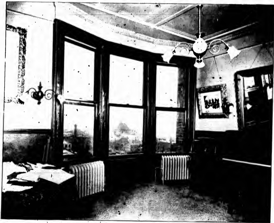
Fig. 149. —Interior View, Temple Building, Toronto.
