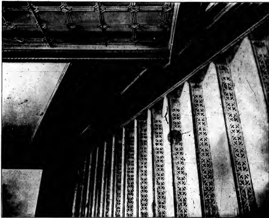
Fig. 148. Interior View, Temple Building, Toronto.
