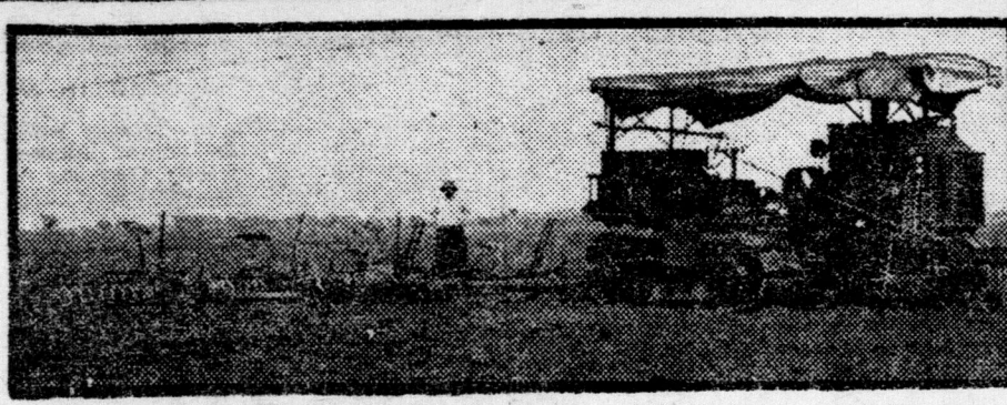
The Caterpillar Tractor, which takes place of forty horses and ten men on B. F. Bradley's Fertile Meadow Farm. A search light is used at night, enabling the tractor to work twenty-four hours. In the above picture the tractor is haul- ing five four-horse discs.
