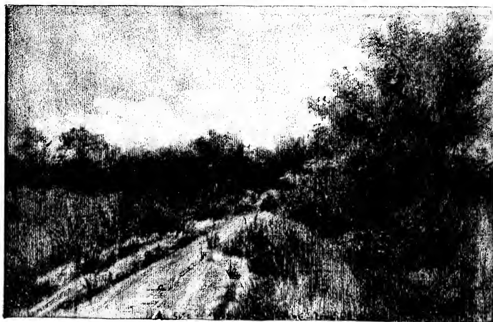
SITE OF WOMAN'S AND FISHERIES BUILDINGS BEFORE GROUND WAS BROKEN.
