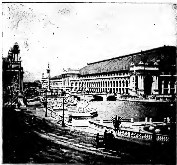
WEST SIDE OF MANUFACTURES AND LIBERAL ARTS BUILDING.
