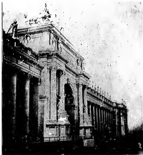
EAST SIDE OF PERISTYLE, LOOKING NORTH.
