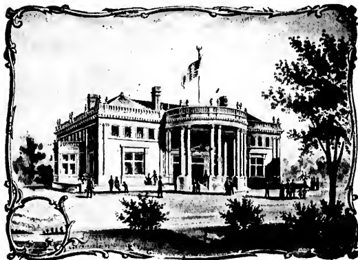
OH O BUILDING.
