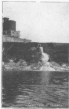
Cut No. 31 Sulphite Mill discharging directly into river
