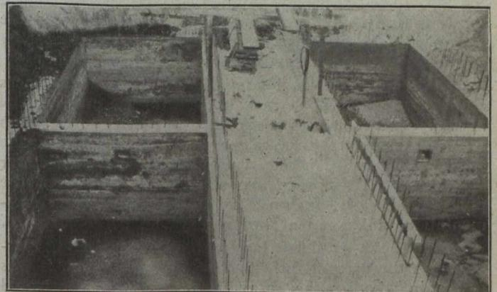
Sedimentation Tanks, Showing Lower Sections.
