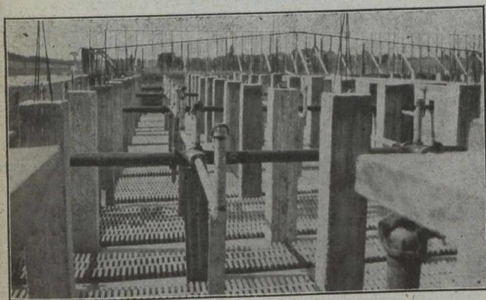
**Interior of Filters, Showing Brick, Piers, Piping and Forms for Siphon and Dosing Chambers.**
