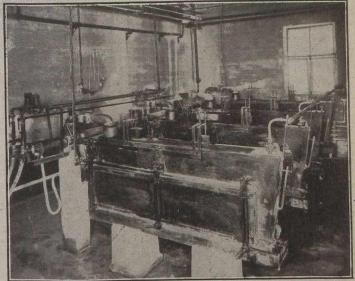
View Showing the Four Electrolytic Cells in Use.
