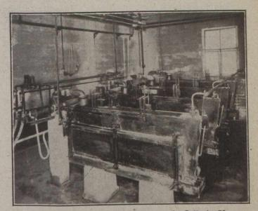
View Showing the Four Electrolytic Cells in Use.
