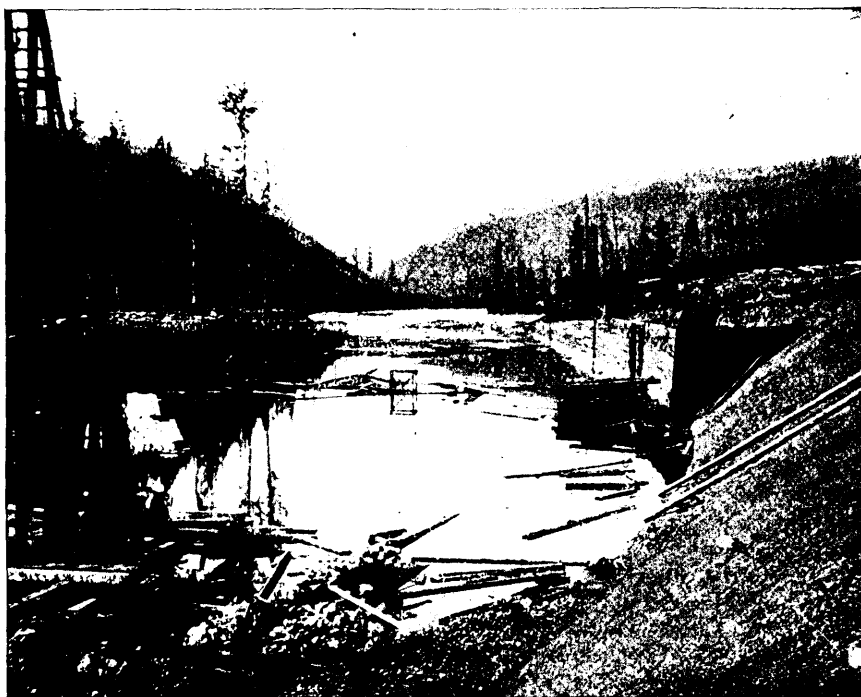
GOLDEN RIVER QUESNELLE CO.'S ENTERPRISE—DAM UNDER CONSTRUCTION. (From a photo taken last year).
