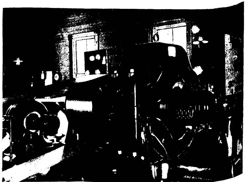
FIG. 3.—POWER GENERATOR AND ALTERNATOR.
