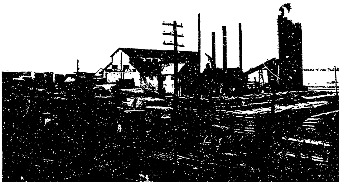
View of Saw Mill, East Side
