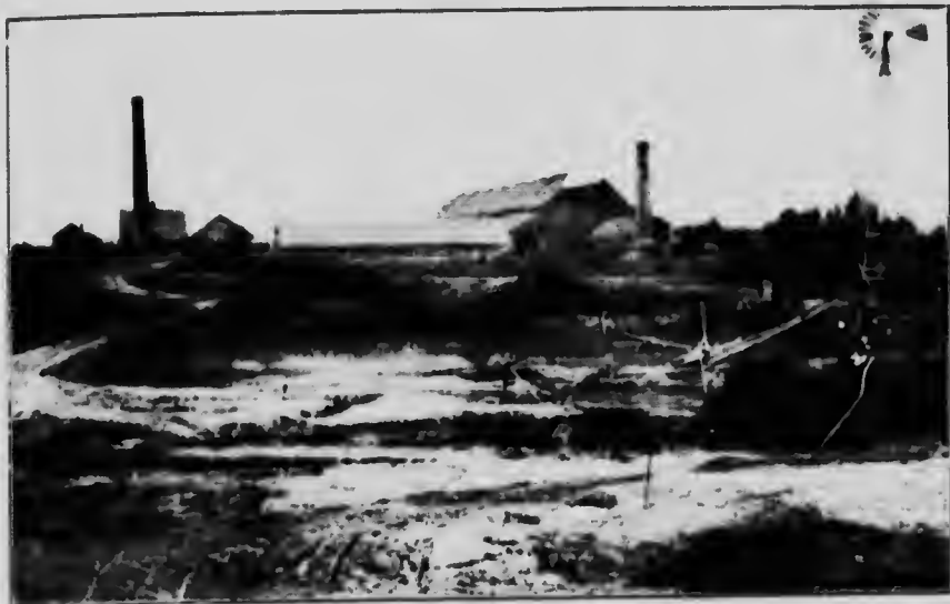
Robert Shaw's brick works, Avonport, Nova Scotia.
