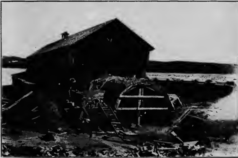
Continuous kiln under construction, Mira River Brick Co., Cape Breton.
