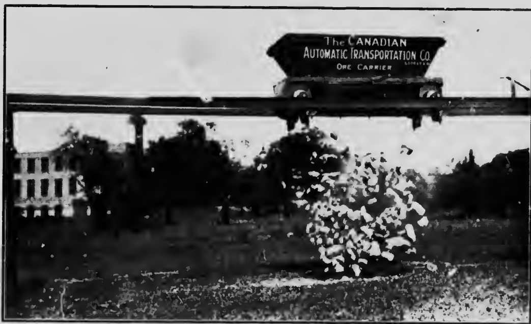
ELECTRIC CARRIER AUTOMATICALLY DUMPING ORE
