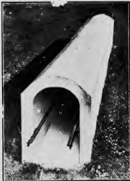
SECTION CONCRETE TUBE UNDERGROUND SYSTEM
