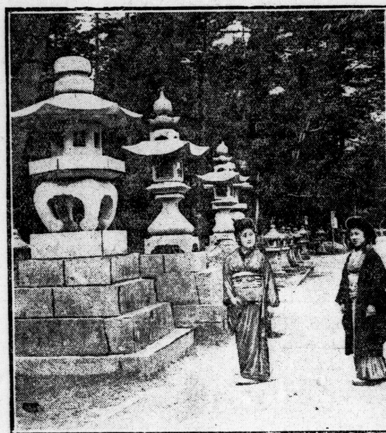
Picturesque street lights are seen in some parts of Japan. On the right are rows of stone lanterns to light the pathway.
