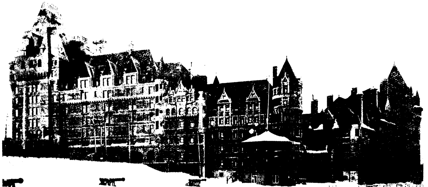
New addition Chateau Frontenac, Quebec, built, KAHN SYSTEM concrete reinforcement. W. S. Painter, architect; Canadian Stewart Co., Montreal, contractors.
