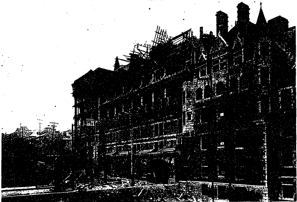
NEW ADDITION TO CHATEAU FRONTENAC, QUEBEC CITY. VIEW TAKEN OCTOBER 1ST, SHOWING THE EXTERIOR OF THE LOWER PORTION OF THE BUILDING FINISHED, AND THE FORM WORK OF THE ROOF IN COURSE OF PREPARATION. NOTE THE MANNER OF MAKING THE CONNECTION BETWEEN THE OLD AND NEW PART, THE GENERAL TREATMENT EFFECTING A PERFECT ASSIMILATION. W. S. PAINTER, ARCHITECT.
