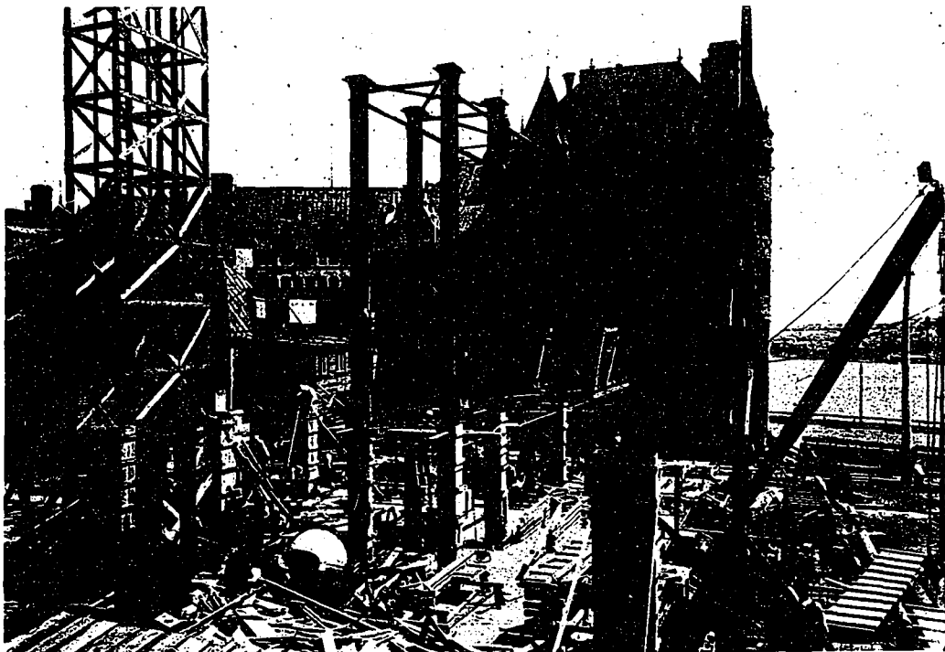
NEW ADDITION TO CHATEAU FRONTENAC, QUEBEC CITY. VIEW SHOWING THE TEN STRUCTURAL STEEL COLUMNS AND STEEL TRUSSES USED IN THE BUILDING, AND THE PROGRESS OF THE WORK MADE UP TO JULY 22ND. W. S. PAINTER. ARCHITECT.
