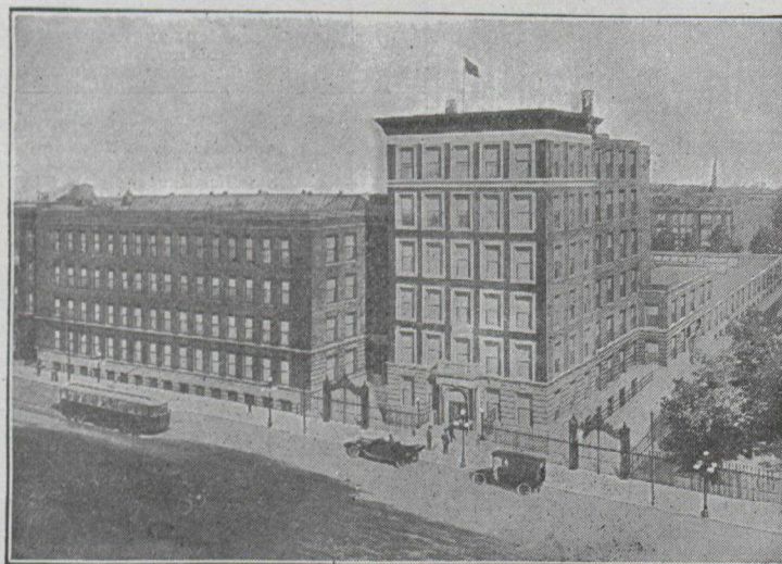
FIRE PROOF BUILDINGS
