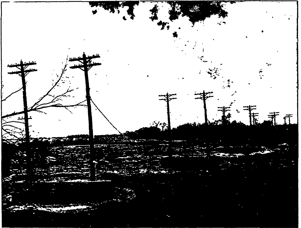
FIG. 7.—POLE LINE OVER RICHELIEU RIVER.
