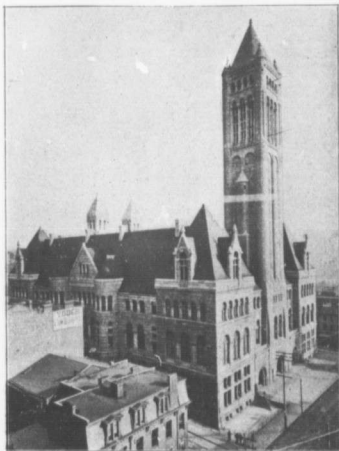
Allegheny County Court House, Pittsburgh.
