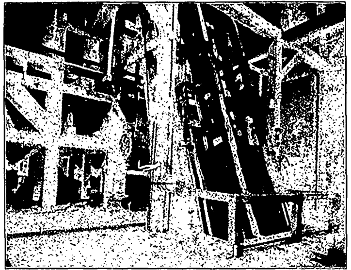
Shaft at Surface, Centre Star.
