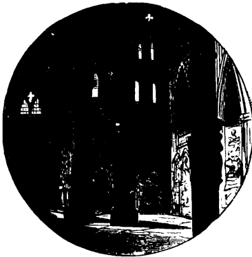
INTERIOR OF CANTERBURY CATHEDRAL.
