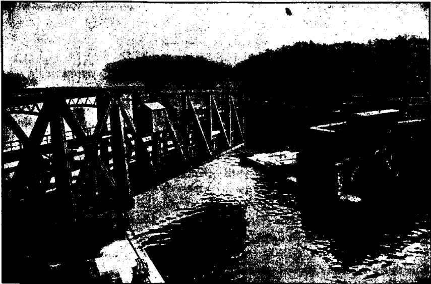
AQUEDUCT BEING SWUNG ASIDE TO ALLOW VESSEL TO PASS ON SHIP CANAL BENEATH
