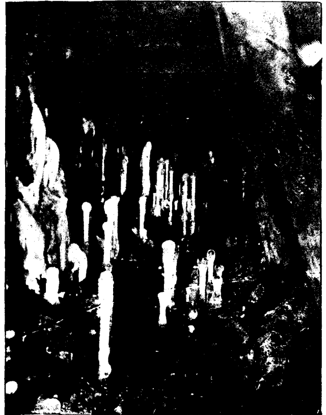
A Tunnel in the Nickel Plate, showing curious formation of "Inverted Icicles" from Water dripping from the Roof in cold weather.
