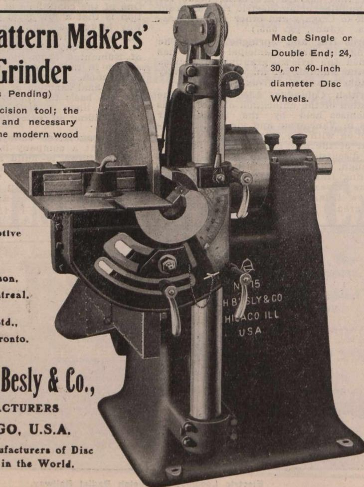
Made Single or Double End; 24, 30, or 40-inch diameter Disc Wheels.
