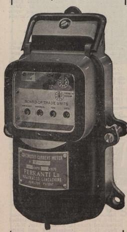
The guaranteed accuracy of the Ferranti Traction Meter is 21/2 per cent. from full load to 1-10th load.
