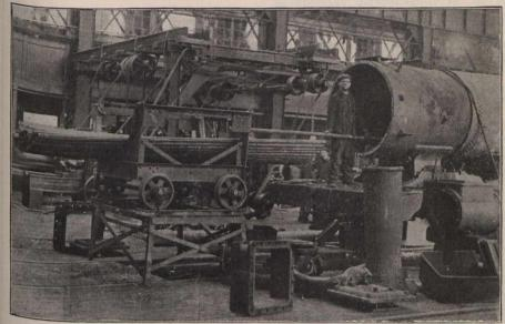
Fig. 1. Removing Tubes from Boiler for Putting on New Ends.
