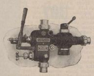
Lifting Locomotive Injector is a self-adjusting and re-starting instrument designed to meet modern locomotive conditions. It will feed water at a higher temperature than ordinary service demands, and the delivering capacity increases with increasing pressure.
