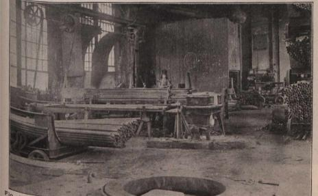
Fig. 4. Department where the Tubes are trimmed, New Ends welded on, and finally cut to Length.
