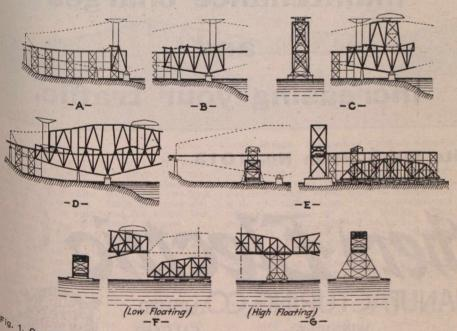
Fig. 1. Quebec Bridge. Scheme of erection, St. Lawrence Bridge Co.'s designs A, B and X.
