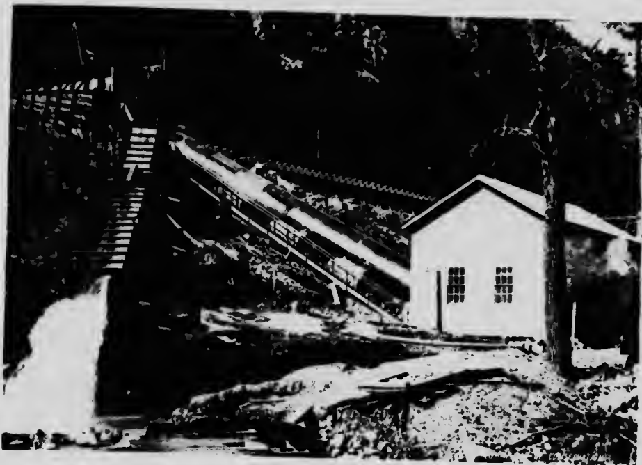
SIMILKAMEEN RIVER POWER PLANT OF THE DALY REDUCTION CO. Showing forebay, steel penstock and power house. Head developed, 67 feet. Hodley, B. C.
