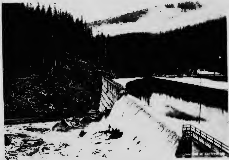
BRITISH COLUMBIA ELECTRIC RAILWAY CO. Ambursen type of dam on Jordan river, Vancouver Island, with water passing over spillway.
