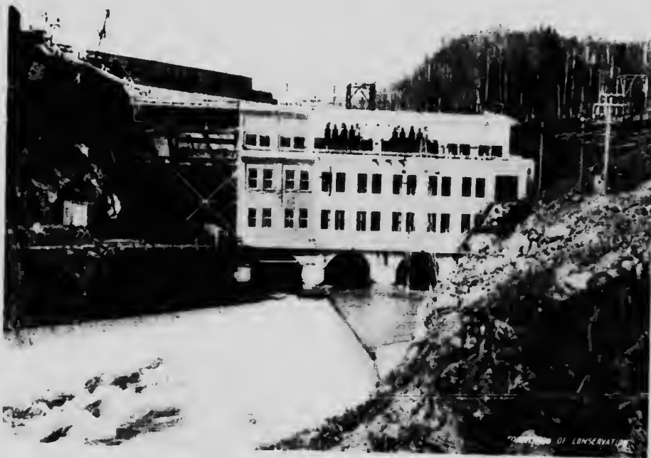
WESTERN CANADA POWER CO STAVE FALLS DEVELOPMENT
