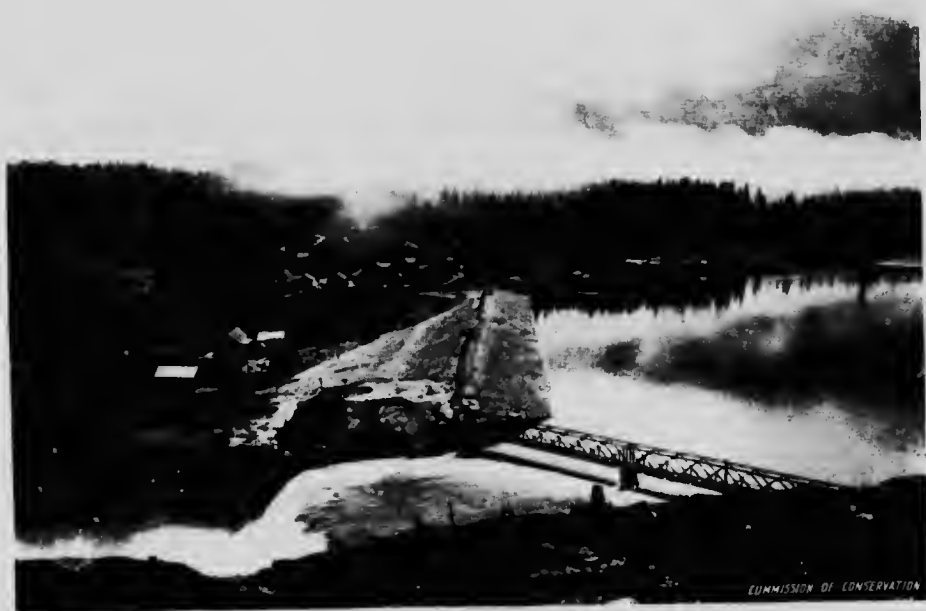
BRITISH COLUMBIA ELECTRIC RAILWAY CO. Coquitlam-Buntzen development General view of Coquitlam hydraulic-fill dam with water flowing over spillway.
