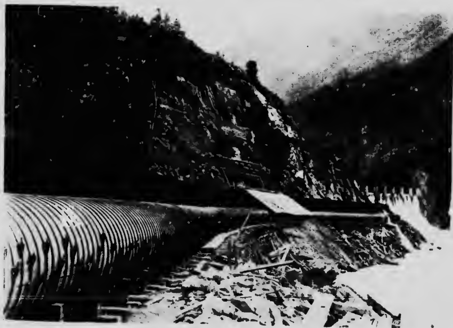
REVELSTOKE HYDRO-ELECTRIC DEVELOPMENT, ILLECILLEWAET RIVER Showing in-take dam and wood stove pipelines. Canadian Pacific Ry. grade may be seen above.
