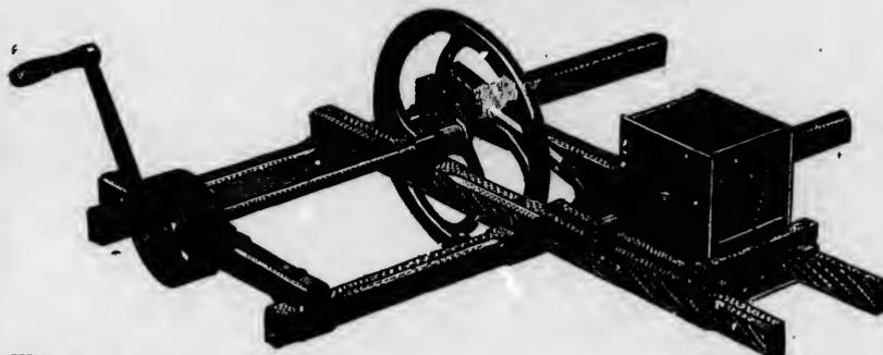
Will cut the toughest curd as thoroughly as the tenderest and is therefore adapted to any kind of curd. When run by steam power it will cut as fast as one man can feed it
