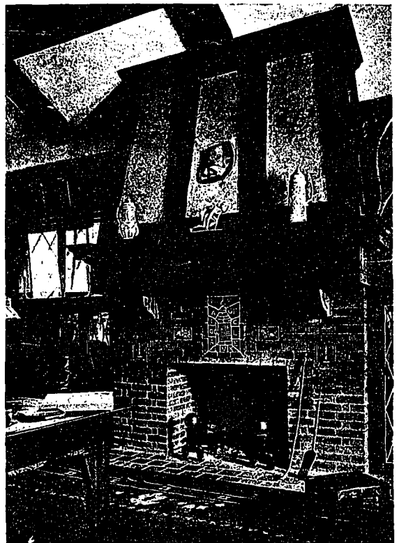
Fireplace in Living Room, Residence of Frederick Paul, Castle Frank Road, Toronto. The Bricks Vary from Brown to Red, and the Hearth is Laid with Red Welch Pavers. Note the Crane and Sturdy Character of the Heavy Wrought Iron Fire-Dogs. Langley and Howland, Architects.
