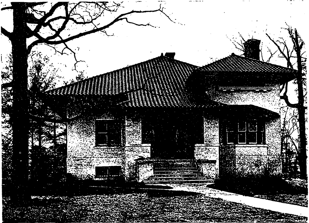
This View Shows the Main Approach and the Heavy Oak Entrance Door, Hung on Wrought Iron Strap Hinges. The Walls are of Hard Brick, Plastered on the Exterior With a Roughcast Cement; the Roof is of Red Unglazed Spanish Tile, and the Windows Throughout are of Polished Plate Glass with Small Diamond Panes in the Upper Sash. Langley and Howland, Architects.
