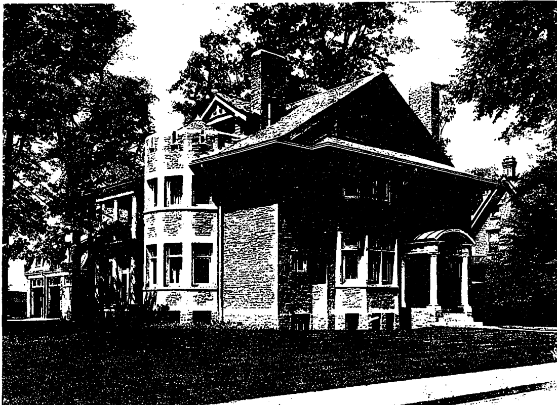
Residence of Mrs. C. C. Cummings, Corner of Hawthorne and Dale Avenues. A Modern House in Character of the Old English Type, Set on a Spacious Site and Built of Credit Valley Random Rubble. J. A. McKenzie, Architect.
