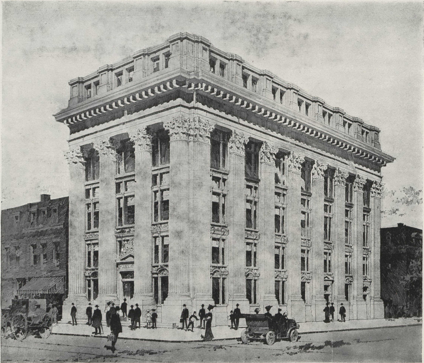
Bank of Toronto, St. Catherine St. Branch, Montreal. Messrs. E. & W. S. Maxwell, Architects. Walter Ryan, Plumber.
