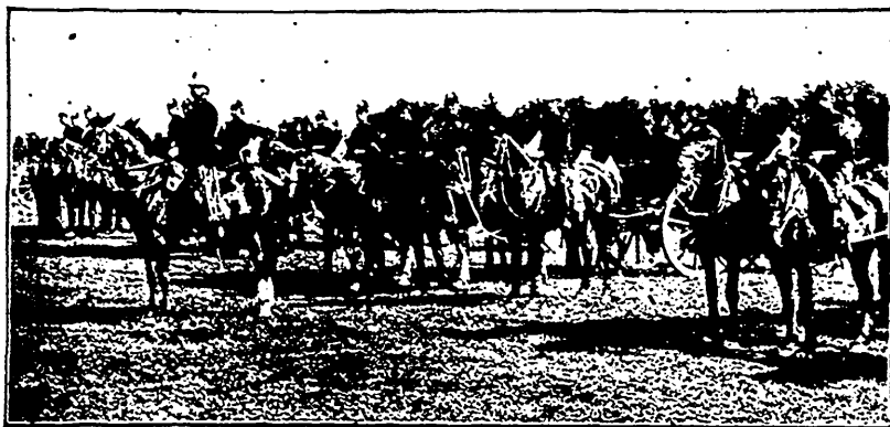
FIELD BATTERY IN QUARTER COLUMN.
