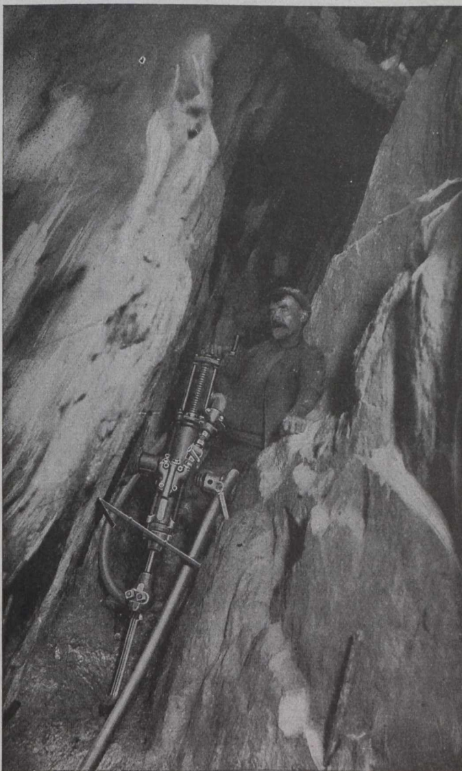
A Piston Drill at Work in an 18-inch Stope
