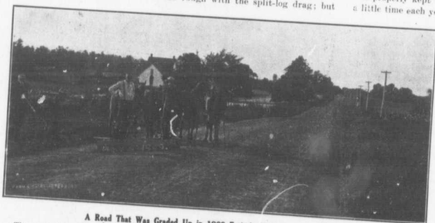
A Road That Was Graded Up in 1909 Entirely With the Split-log Drag The possibilities of the split-log drag are well illustrated in the photo reproduced above. This road in the township of Clinton, near Beamsville, Ont., was turnpiked up from the flat by means of a split-log drag.
