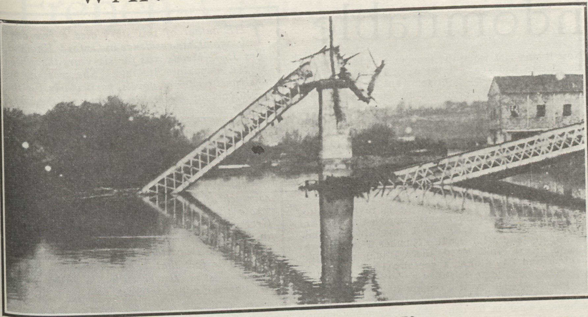
ONE OF MANY DESTROYED BRIDGES.
