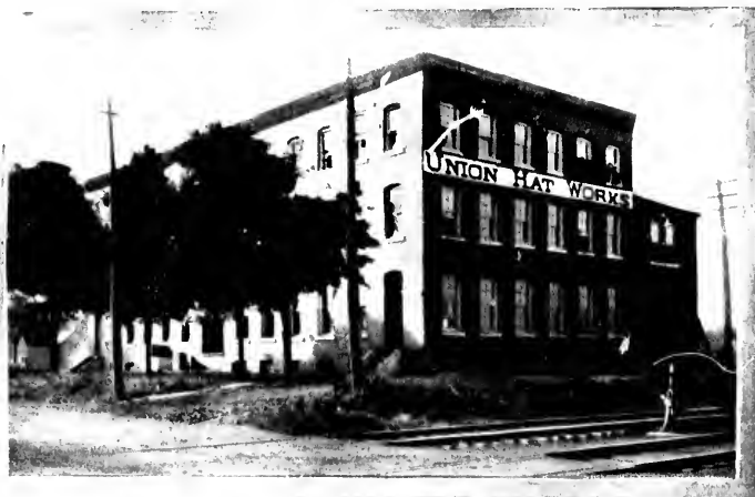
Brockville Hat Works.
