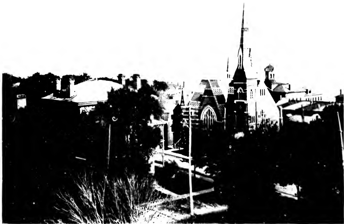
Looking towards River from Court House
