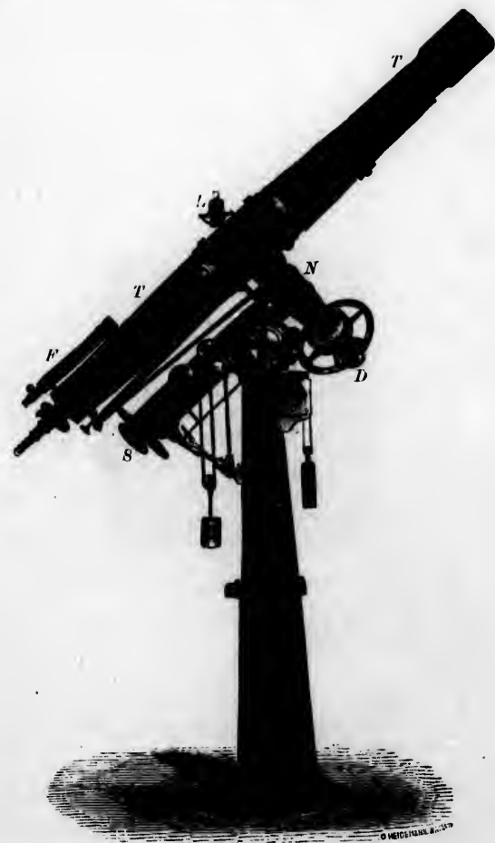
FIG. 37.—EQUATORIAL TELESCOPE POINTED TOWARD THE POLE.
