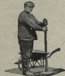
The mixture is well tamped and covered with screenings
