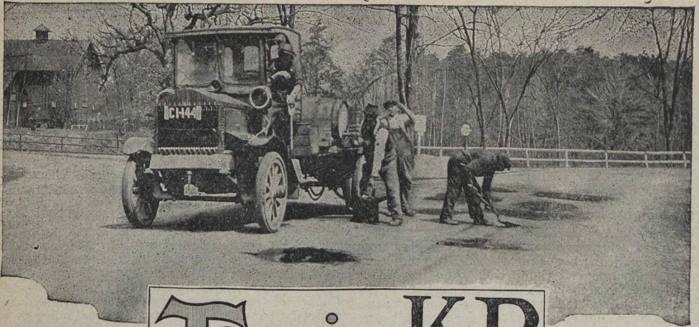
Patrol maintenance crew patching with "Tarvia-KP."
