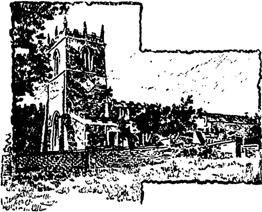
PARISH CHURCH, EPWORTH.
