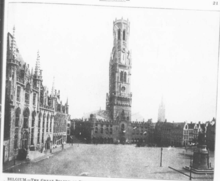
BELGIUM.—THE GREAT BELFRY AT BRUGES.—Two hundred and sixty-seven feet high and a fine specimen of Gothic architecture. The first storey belongs to the original building which was destroyed by fire in 1280. The second storey was built in the 14th and the third in the 15th century. It has a chime of 47 bells. The poet Longfellow has immortalized these chimes—he stayed awake all night with a "wild delight" listening to them.
