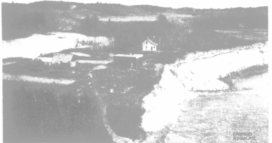
LIGHT AND POWER PLANT ON RED DEER RIVER. SOURCE OF LACOMBE'S LIGHT.
