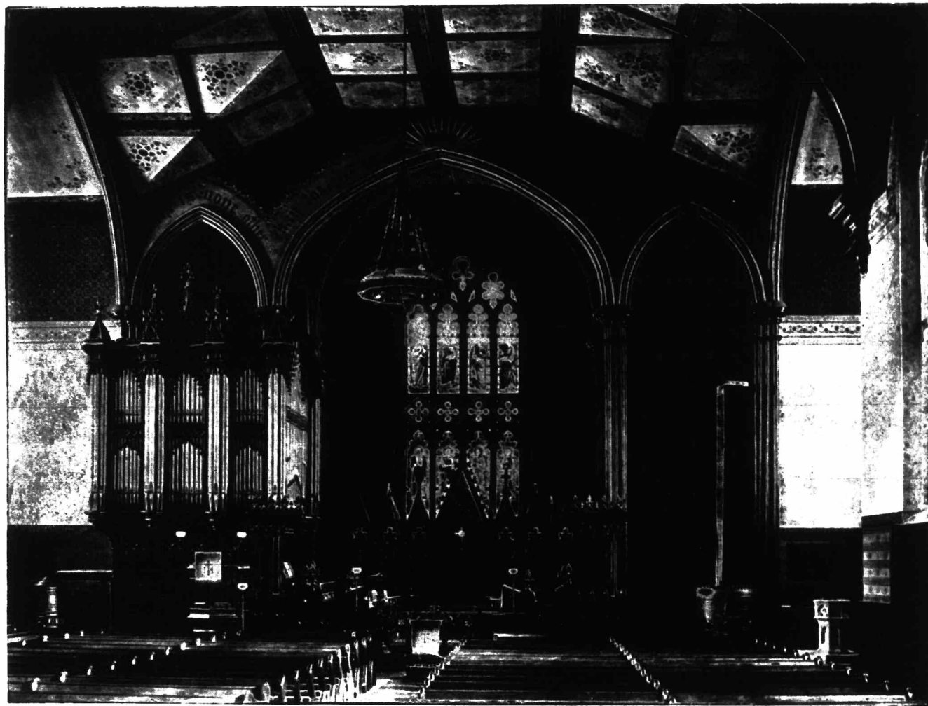
INTERIOR VIEW, HOLY TRINITY CHURCH, TORONTO.
