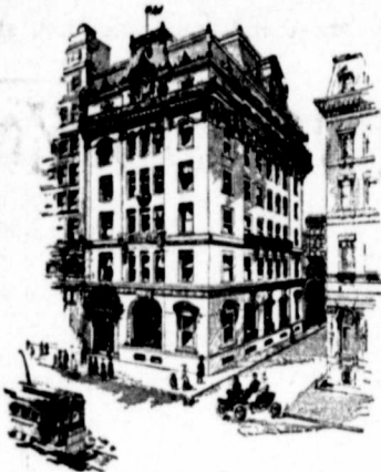
CANADIAN BRANCH LONDON & LANCASHIRE LIFE HEAD OFFICE BUILDING, 77, MONTREAL B. HAL BROWN, GENERAL MANAGER.
