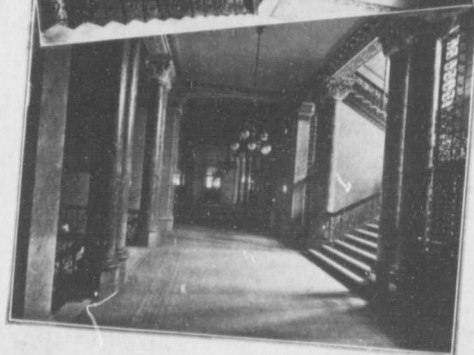
INTERIOR VIEWS OF CITY HALL
