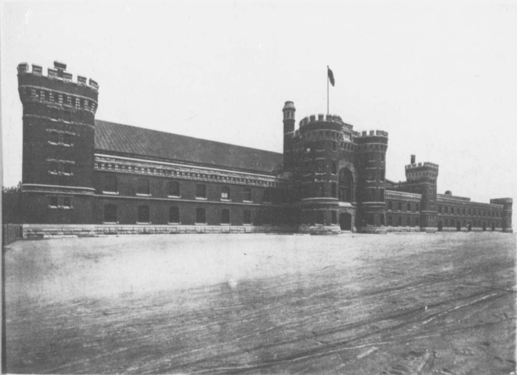
ARMOURIES, SOUTH VIEW
