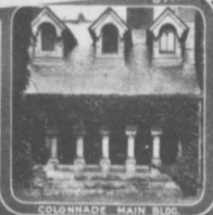
COLONNADE MAIN BLOC
