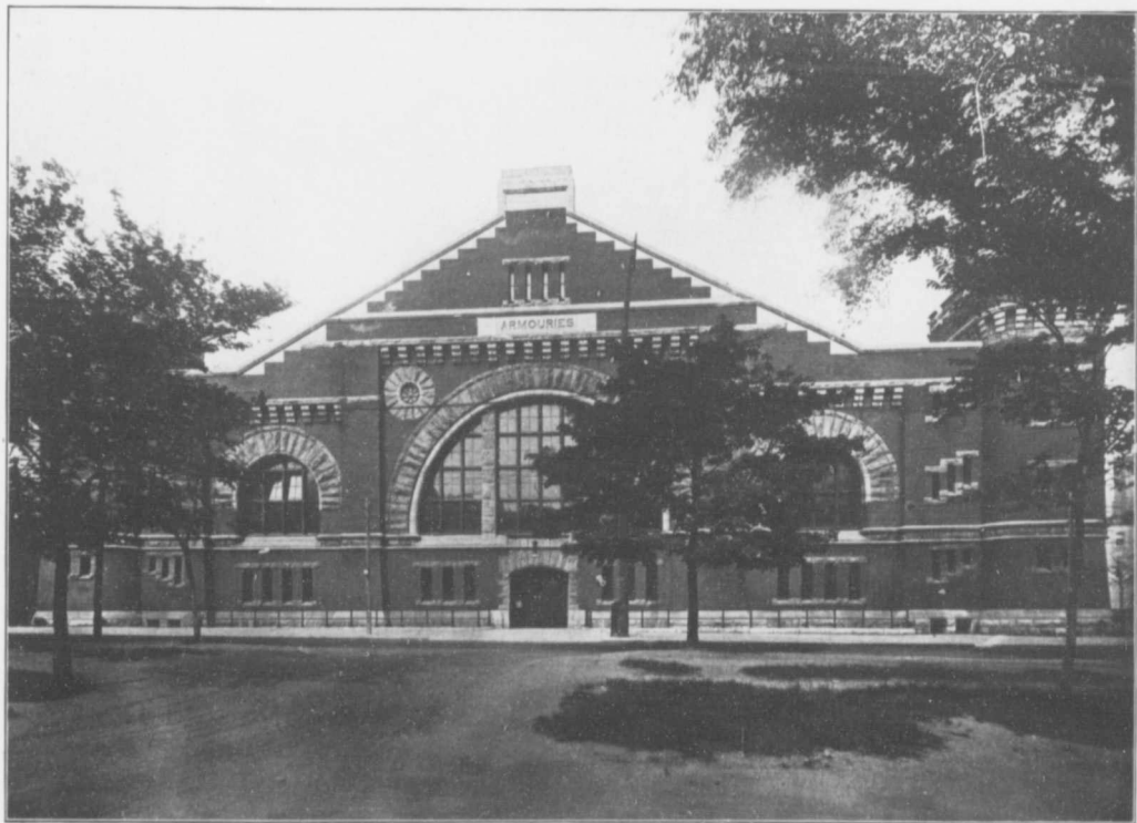
ARMOURIES, FRONT VIEW
