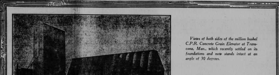
Views of both sides of the million bushel C.P.R. Concrete Grain Elevator at Transcona, Man., which recently settled on its foundations and now stands intact at an angle of 30 degrees.
