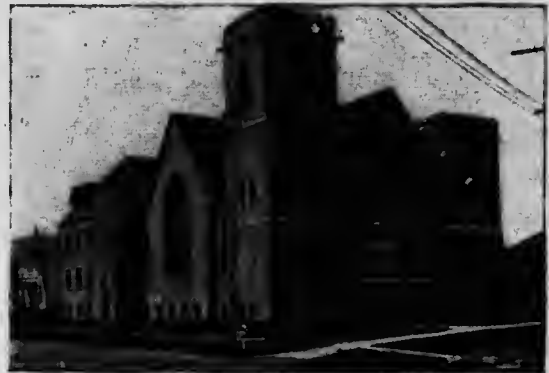
ST. STEPHEN'S CHURCH, WINNIPEG.
