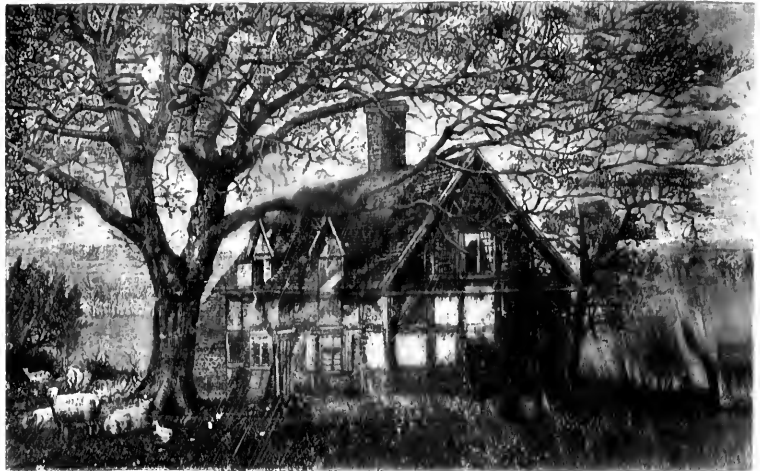
MANWOOD COTTAGE, HANDSWORTH, STAFFORDSHIRE, ENGLAND.
