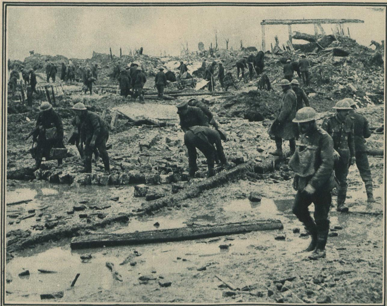
Before the light railways can be laid it is of course necessary to prepare the tracks, and this wherever possible is done along a road. Here Canadian Pioneers are endeavouring to re-make a road which has been battered to bits by shell fire. It is at times almost impossible to say where the road originally ran.
