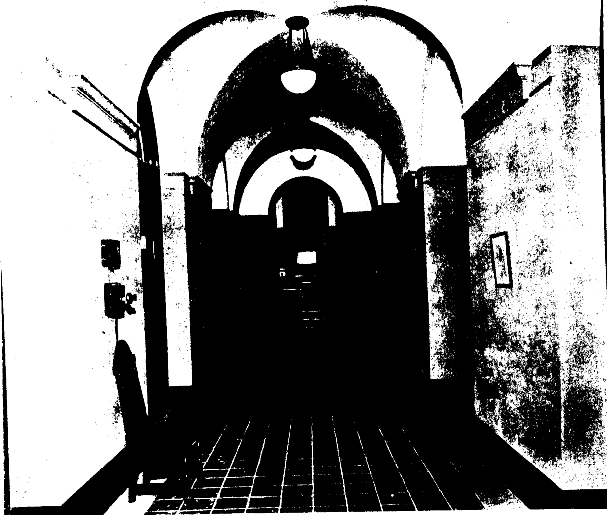
Groined Ceiling in Hallway of Nurses' Home, Toronto General Hospital.
