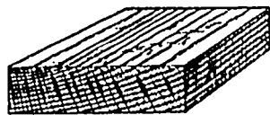
Fig. 5.—“Honeycombed” board. The checks or cracks form along the pith rays
